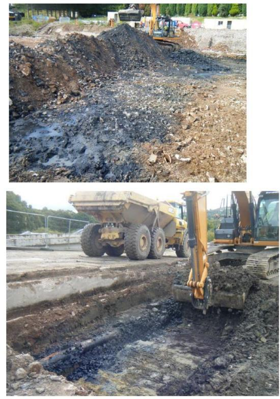
Diggers were able to chase out the contamination and impacted soils were sent off site for disposal.
